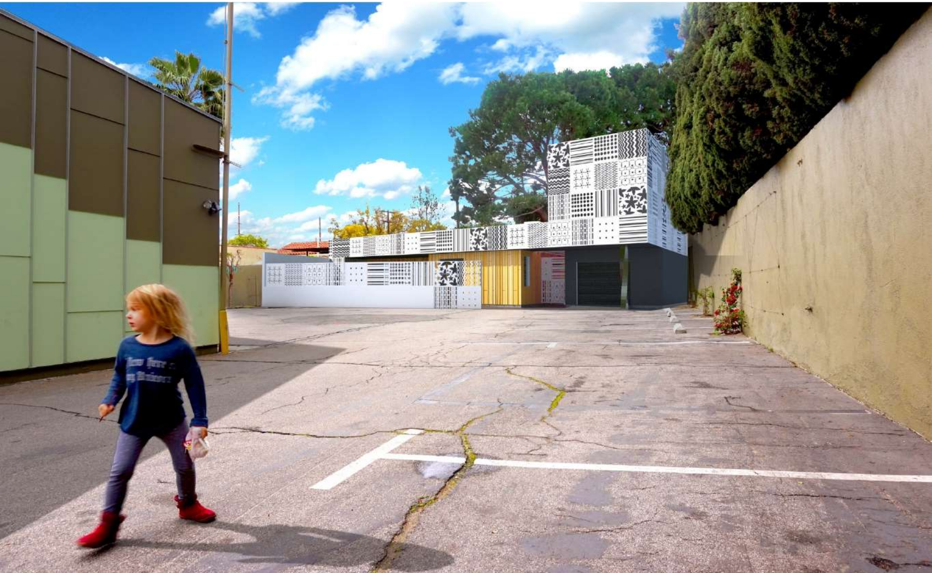
Exterior view: from parking lot
